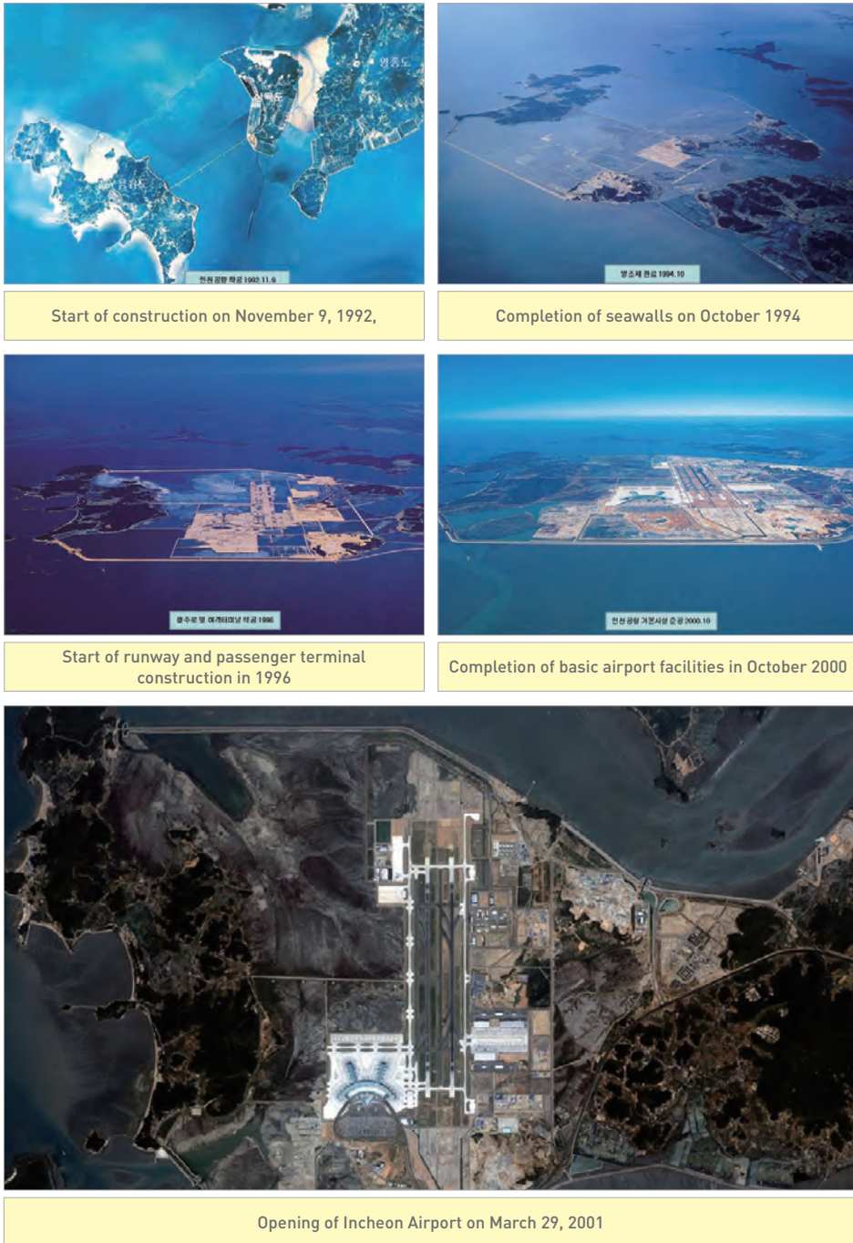
Figure 3.3 Incheon International Airport phase 1 construction process
